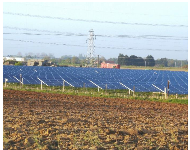
Deepdale Solar Park
