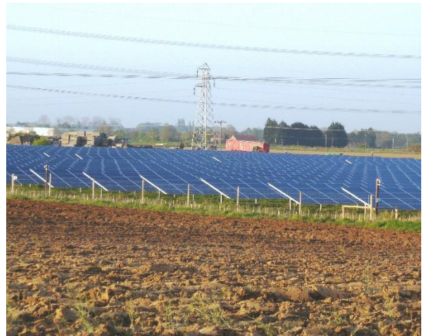
Deepdale Solar Park
