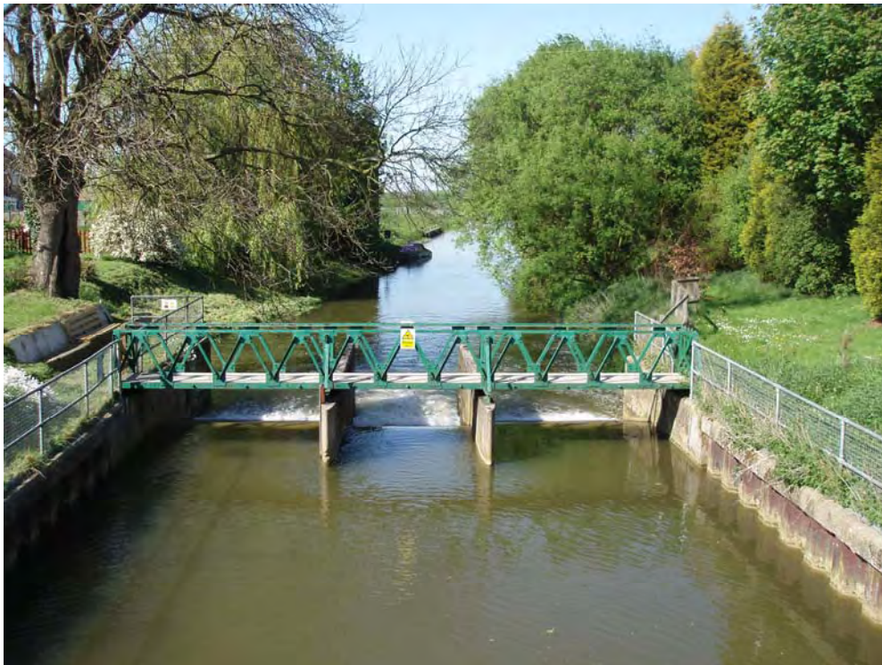
Photograph Gen 15 – River Ancholme View N (downstream) from Bishopsbridge showing flow gauging station.
