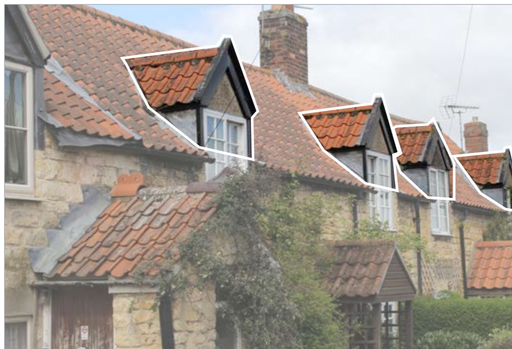
Dormer windows are commonplace in the village core, allowing accommodation in the roof space and helping to reduce building heights.
