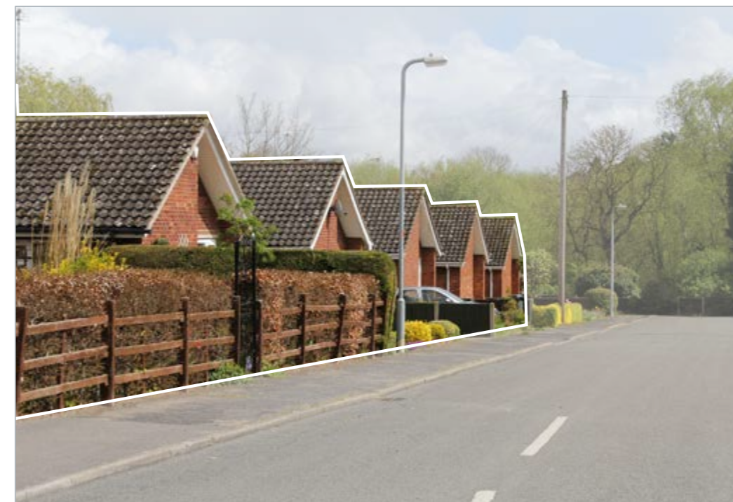
Whilst there is a great deal of variation between buildings, similar buildings are grouped together, creating a consistent character within the street scene.
