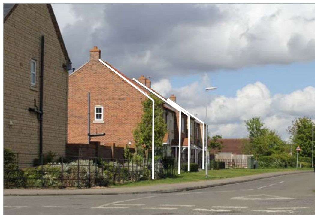
New development on Moor Lane subtly delineates the plot boundary for the terrace by adjusting the building lines.
