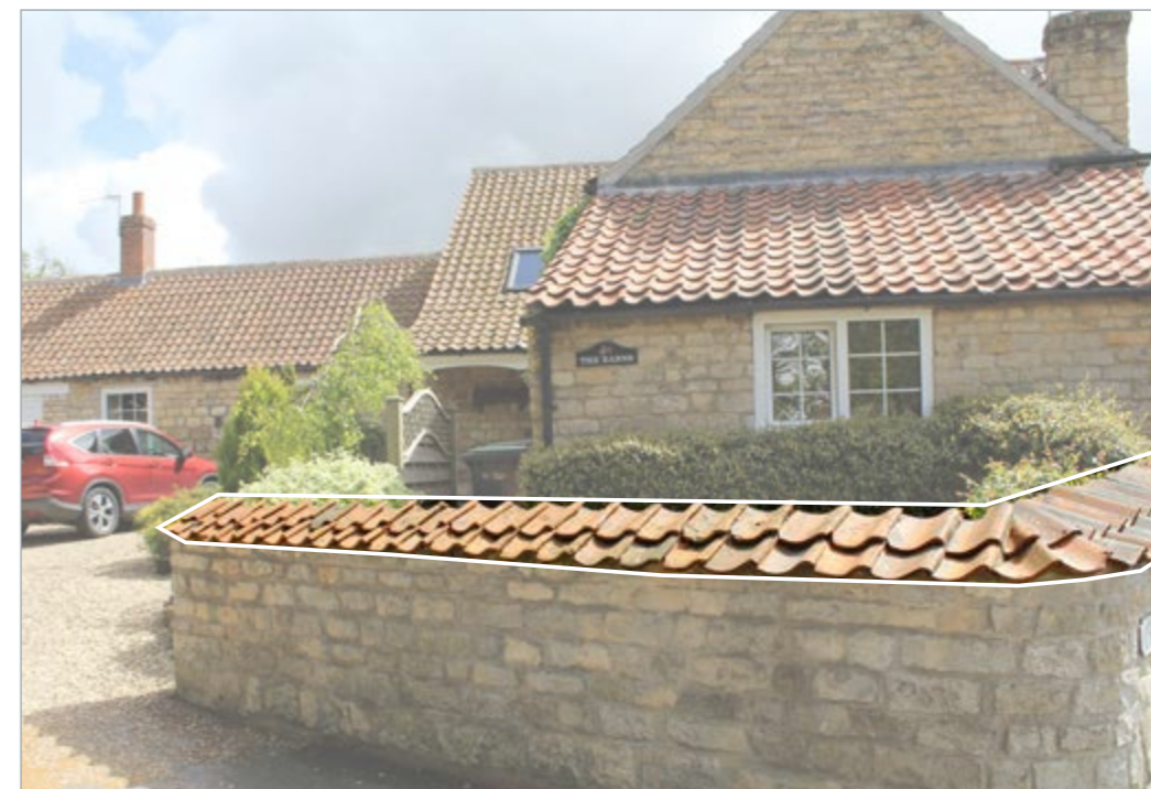
Boundaries are extremely distinctive in the village core, with rubble limestone walls topped with pantile coping.
