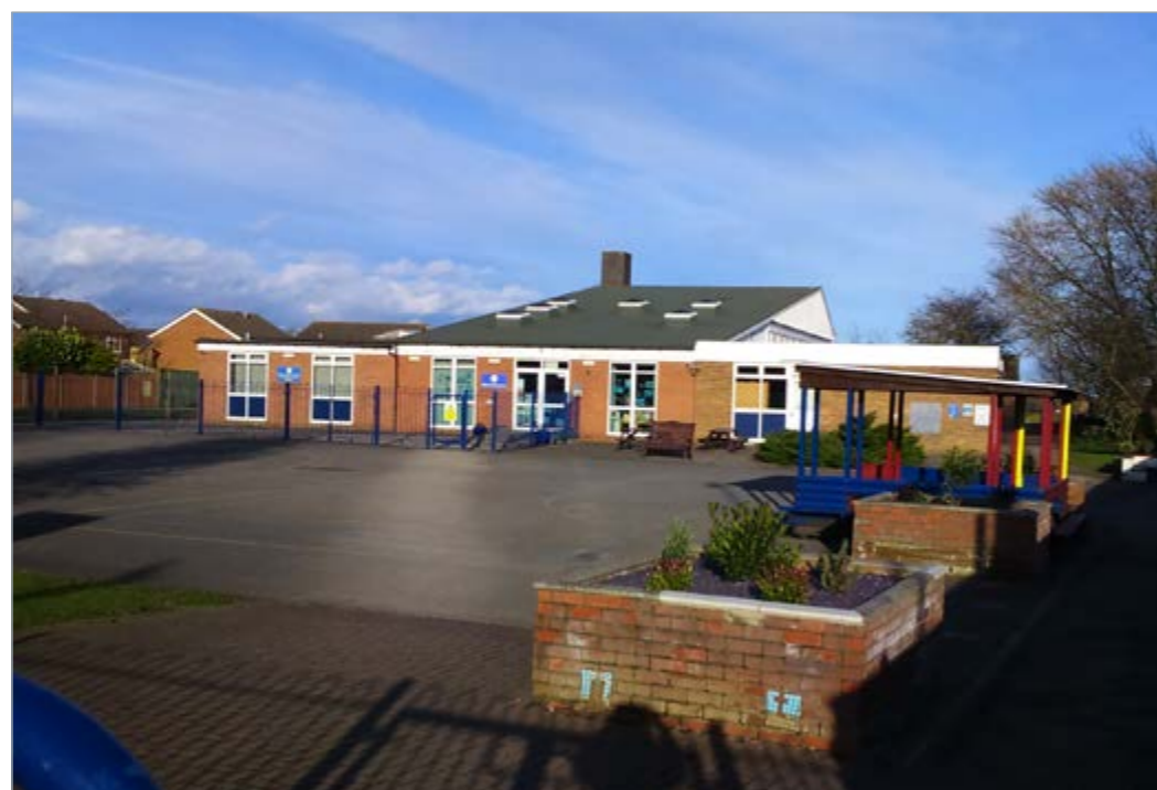
The primary school, located on Station Road.
