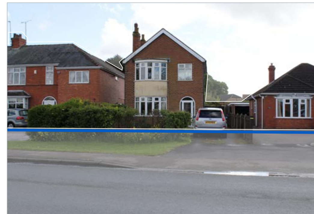
A high degree of differential between plots is present, but a consistent build line helps retain character.
