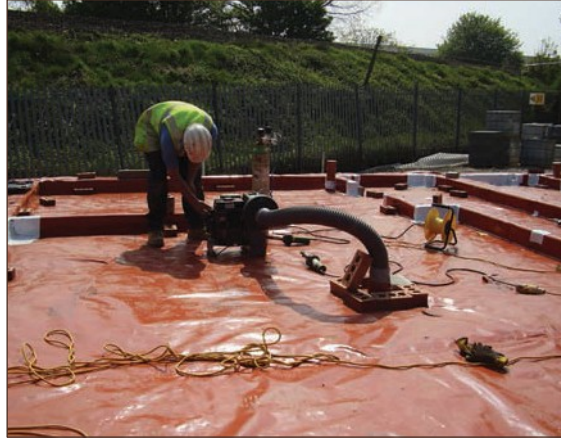
Figure A4.38 Tracer gas testing (courtesy PAGeotechnical Ltd)
