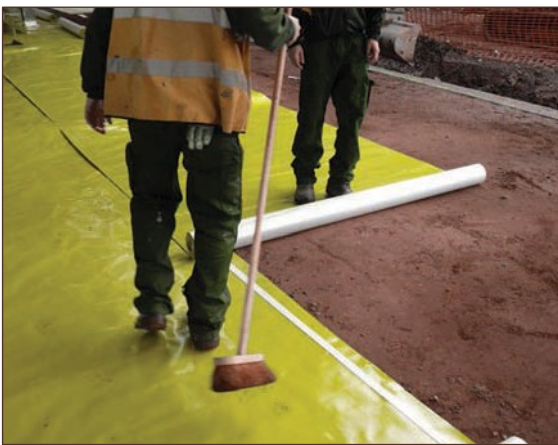
Figure A4.15 LDPE type gas membrane overlap and double sided tape. Sand blinding to protect underside of gas membrane (courtesy A Proctor Group)
