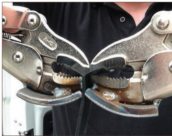
Figure A4.46 Testing a weld with 'dog bone' grips (courtesy MEC Environmental Ltd)
