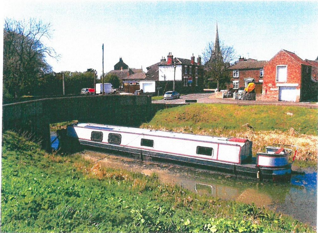
Church Street Bridge Billingham Skirth
