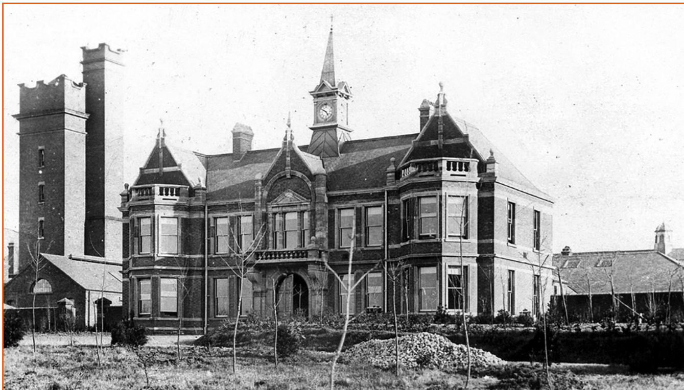
Above: The Administration Block and Water Tower shortly after opening image from www.simoncornwell.com
