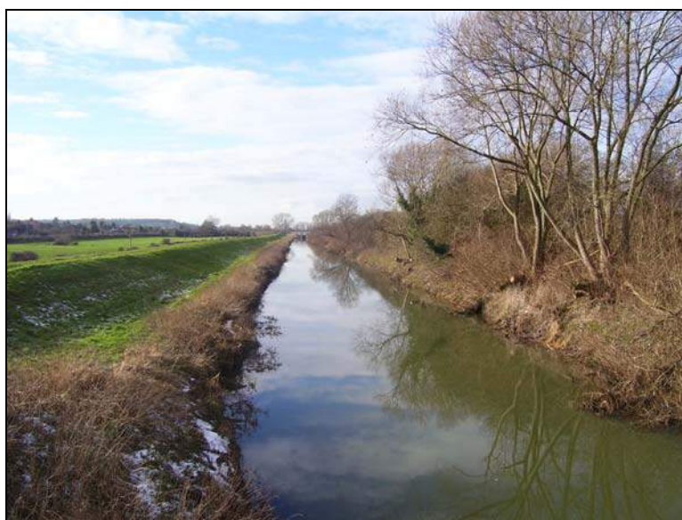
Mill Dam Dyke
