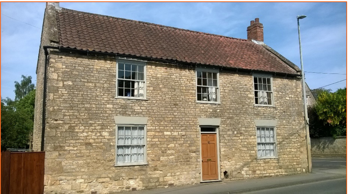
Above: The retention and restoration of original features such as clay pantile roofs and timber windows has a strong positive impact on the conservation area
