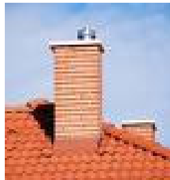
Example of an Internal Chimney
