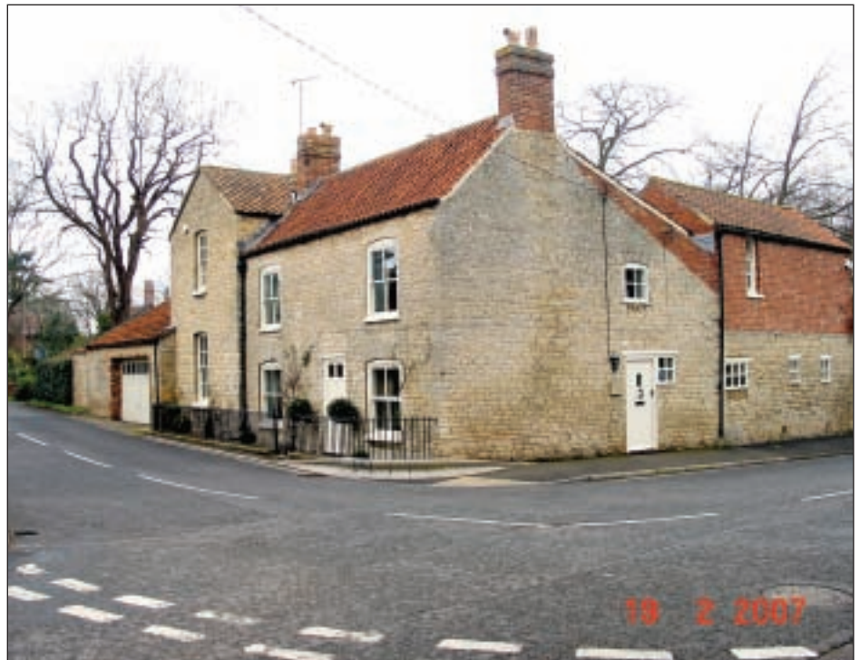
▲ Window openings often have stone heads and cills and are taller than they are wide. Sash windows are common and are set back slightly from the face of the wall. This, together with the step in the centre of the traditional sash windows brings relief to the facades of the buildings. The Stone House, Station Road.
