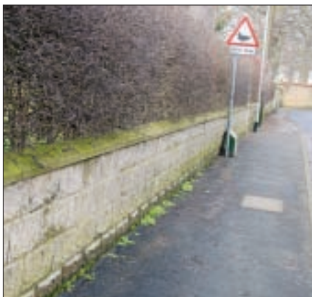
▲ Concrete block wall alongside Mill Lane.
