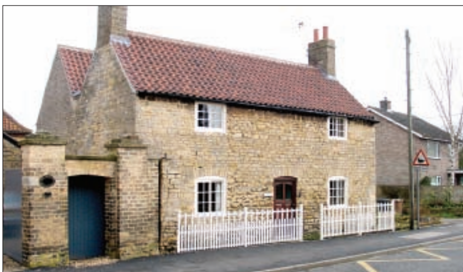
▼ 7 High Street has a mid C18 rear range with an early C19 front range. This elevation has very distinctive Yorkshire sliding sash windows.
