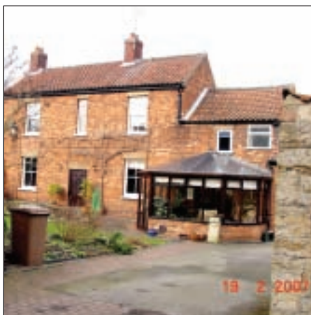
▲ Brick was rare for village buildings until the late C19. This is Little Grange, from Back Lane.
