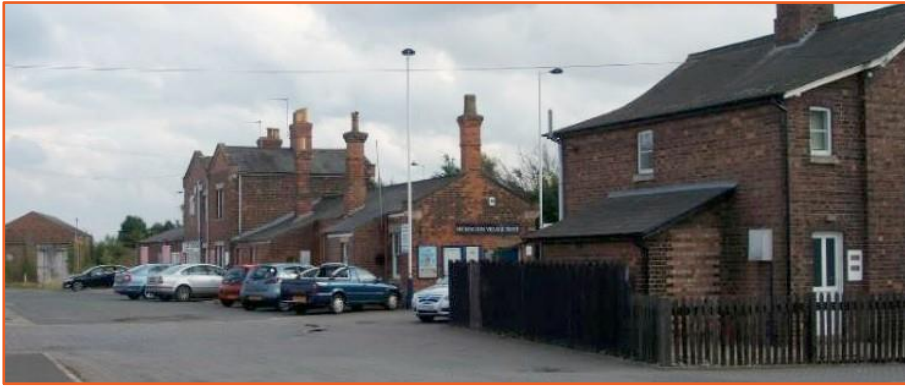
Heckington Station buildings and access
