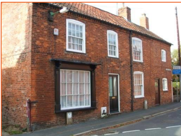
Converted shop front on Church Street
