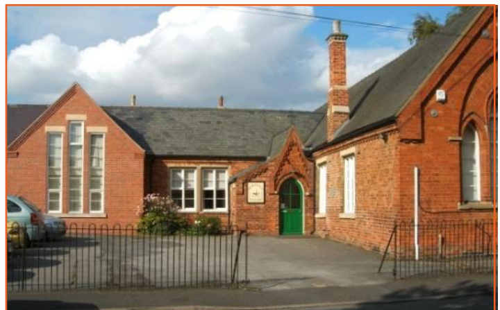
Former school now in use as business premises
