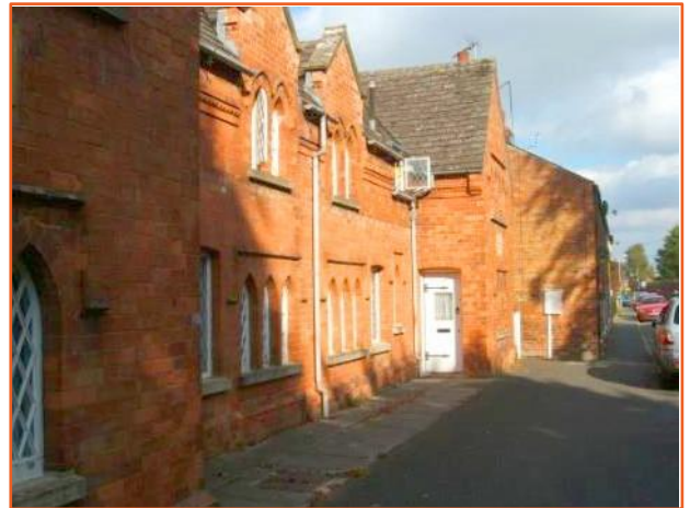
Almshouses on Cameron Street
