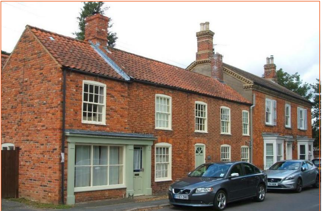
Row of well-maintained buildings on Church Street
