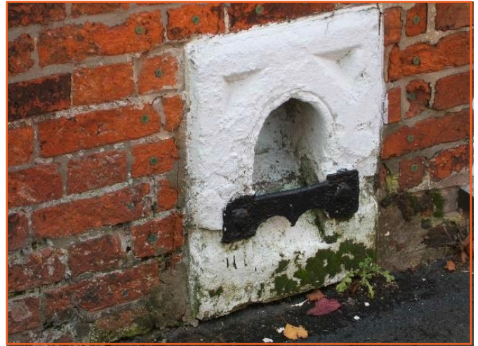
Boot scraper built into a wall on Church St
