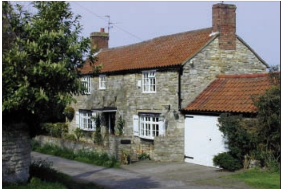
▲ The prevalent local building material up to the middle of the C20 was stone for walls. Buildings have coursed limestone rubble walls and natural clay pantiles on the roof.
