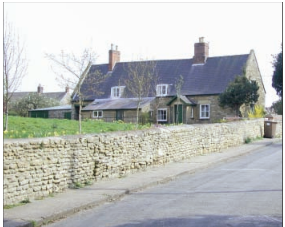
▲ The prevalent local building material up to the middle of the C20 was stone for walls. Buildings have coursed limestone rubble walls and natural clay pantiles on the roof.
