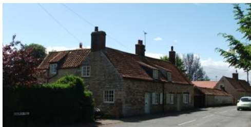
Lincoln Road is host to a row of fine vernacular properties
