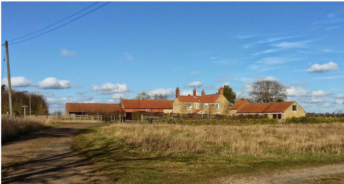
Figure 8 Dunston Pillar Farm
