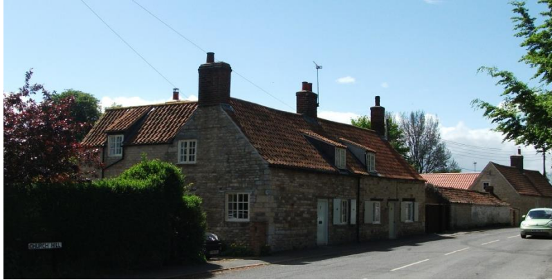
Figure 35: Lincoln Road is host to a row of fine vernacular properties
