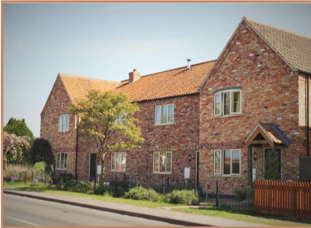
Fig. 28. Photo of the “eco” houses on Walcott Road, highlighting the use of reclaimed brick. (Photo by kind permission of Martin Knowles).
