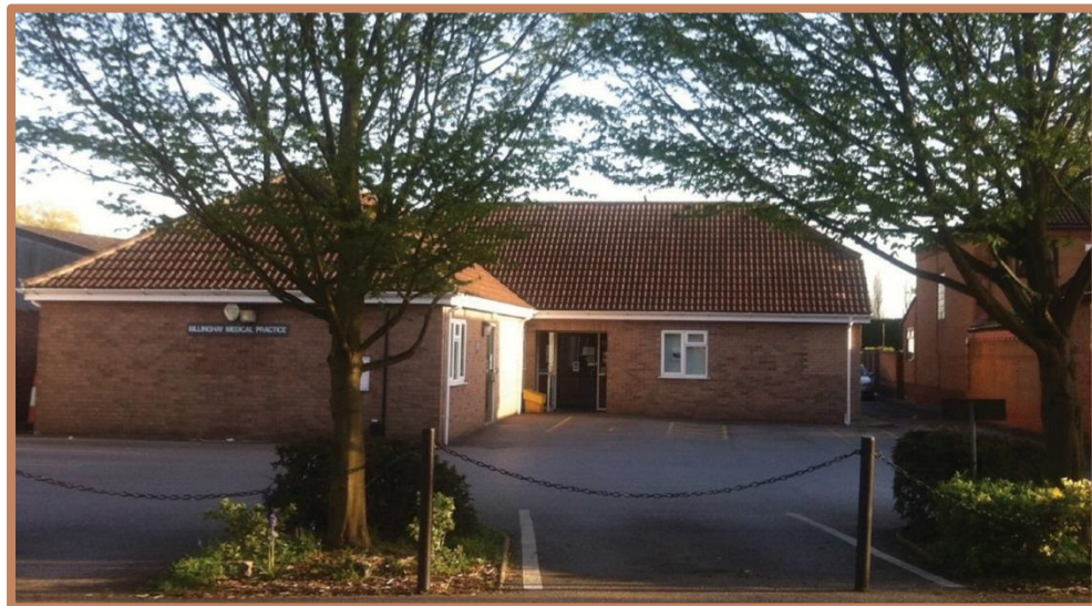
Fig.19. Billingham Medical Centre, dispensary and patient car park.
