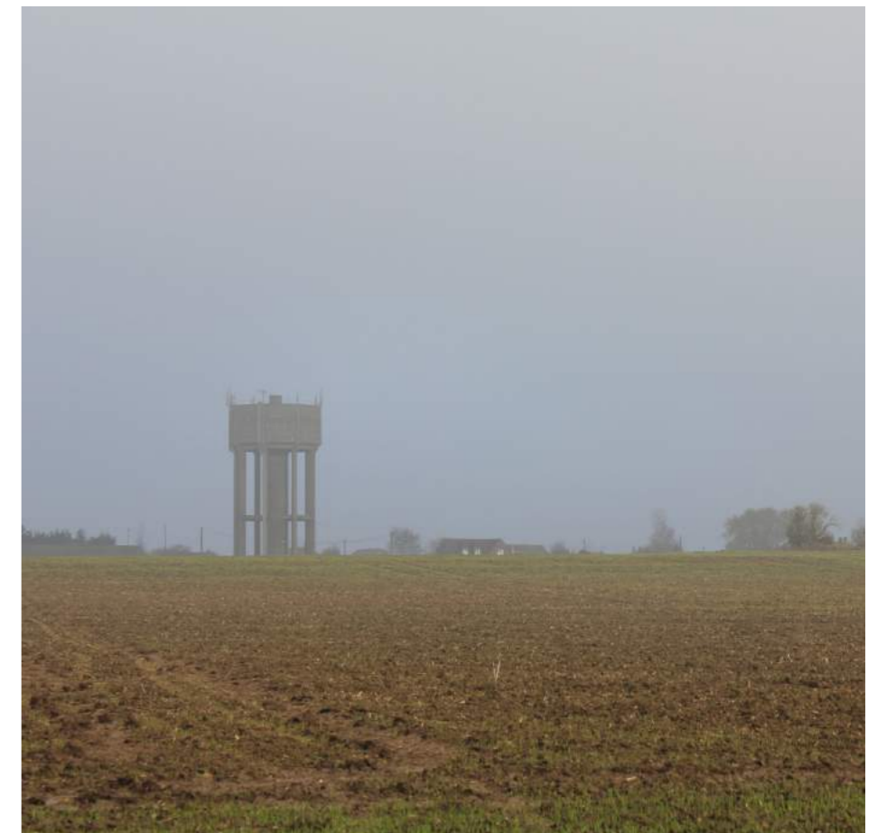
The water tower is a distinctive local landmark
