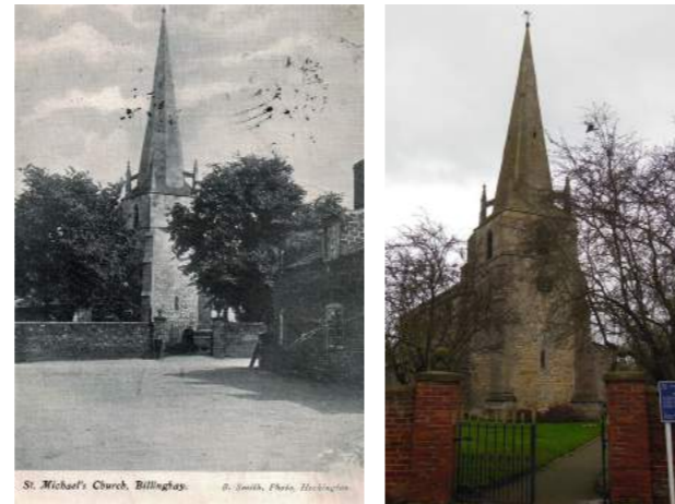
The earliest parts of the Church of St Michael were constructed in the 12th century, with further additions throughout the 13th, 14th and 15th centuries.
