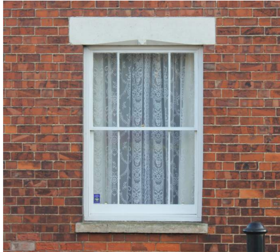
Vernacular red brick buildings with sash windows
