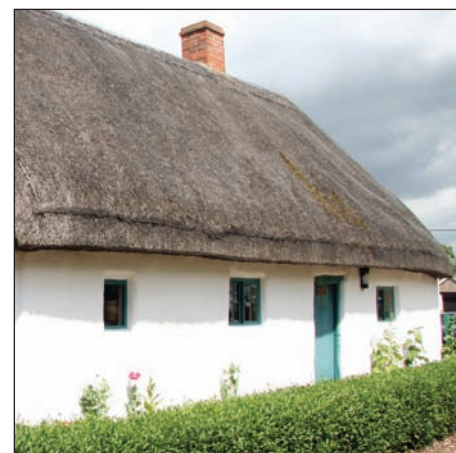
▲ The Old Vicarage is a Grade II listed building and dates from the middle of the C17. The front wall is mud and stud, the traditional Lincolnshire vernacular building material, along with a thatched roof, for cottages of the C16 to C18.
