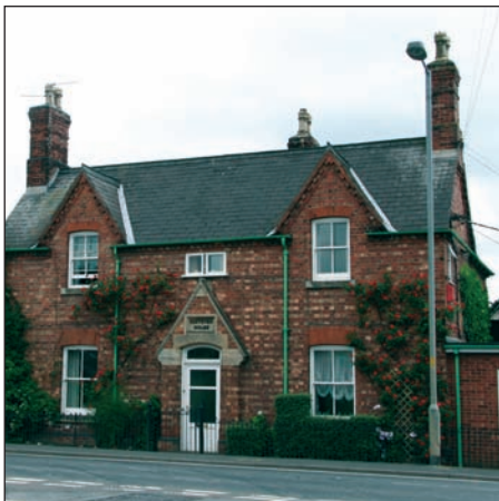
◀ Kesteven House was built as the village Police Station in the late C19.
