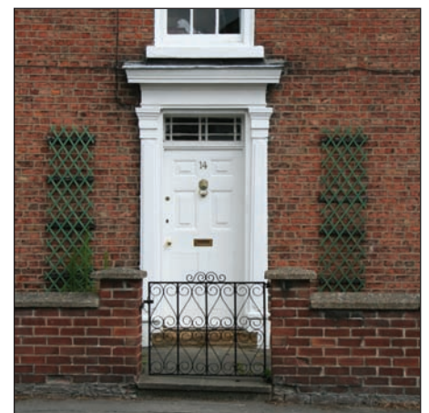
▲ 2765. 14 Bridge Street has a fine entrance door with a margin light fanlight over, a feature typical of buildings of the early C19 in the village.
