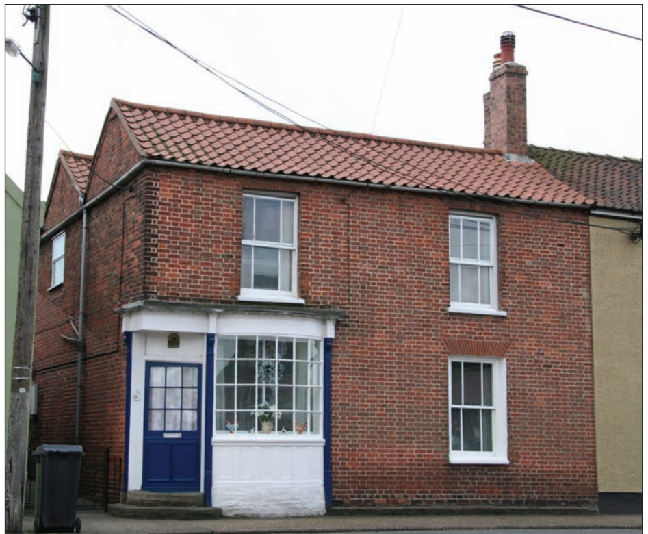
▼ 17 Victoria Street is a Grade II listed building. The corner door to the former shop and the margin light sash windows are typical of the Conservation Area.
