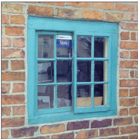
▲ A Yorkshire sliding sash window at The Old Vicarage on Church Street.
