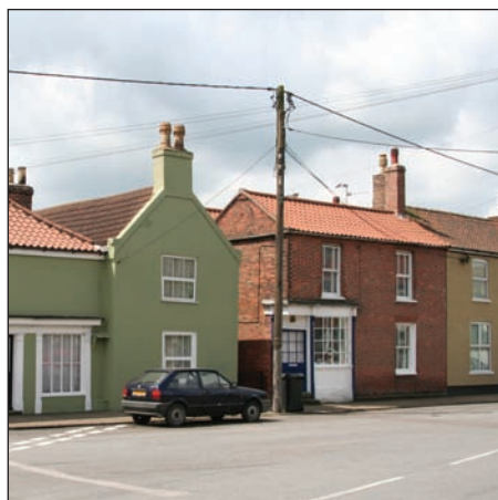
▼ The south side of Victoria Street is lined by buildings dating from the last 200 years.
