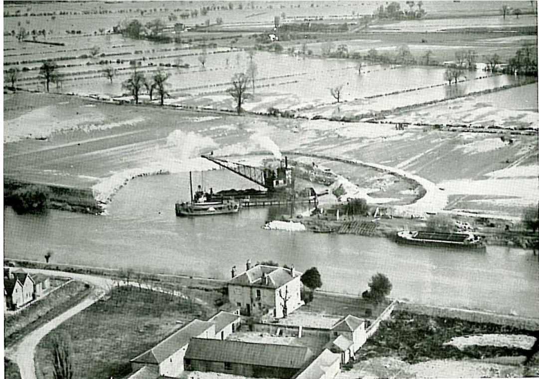
Figure 4.0 – Morton Corner Breach, March 1947.
