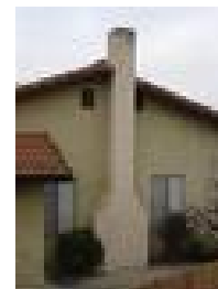
Example of an external Chimney
